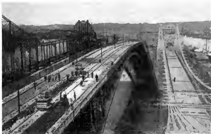
Fig. 4—View showing the Cantilever Railway Bridge, New Steel Arch and Suspension Bridge at St. John, N. B.
